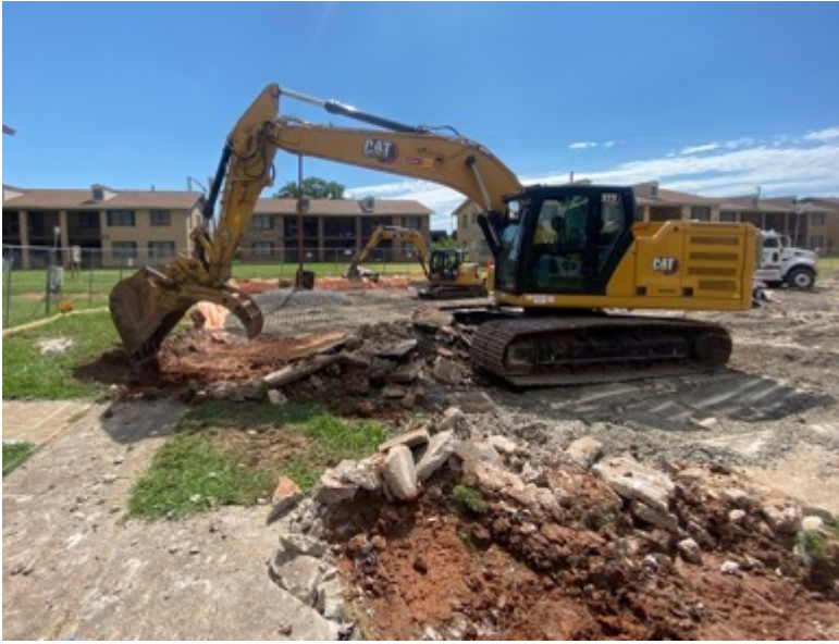
Excavation in north parking lot
