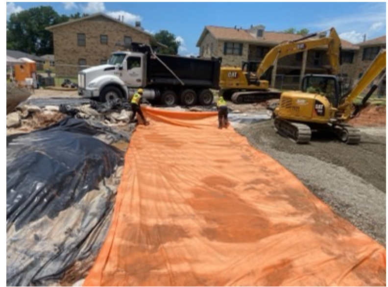
Laying down demarcation fabric after excavation
