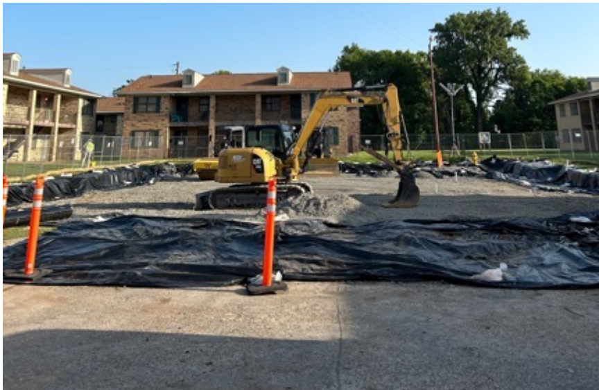
Placing clean backfill
