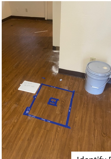
Identify Drilling Locations and Remove Flooring
