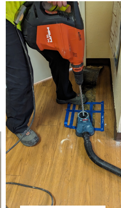
Drill for Sub-Slab Probe Installation
