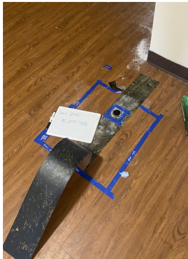
Identify Drilling Locations and Remove Flooring
