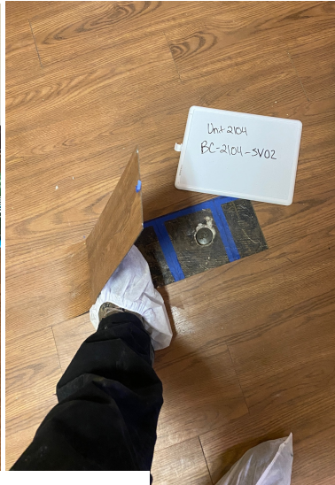
Identify Drilling Locations and Remove Flooring
