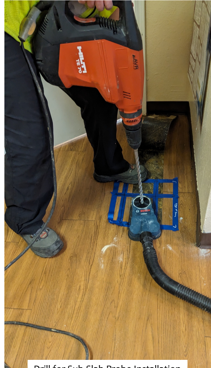
Drill for Sub-Slab Probe Installation
